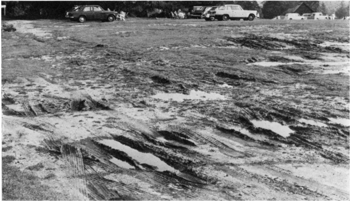
FIGURE 4. Damage done by vehicles on the Open Forest in the 1960s.
