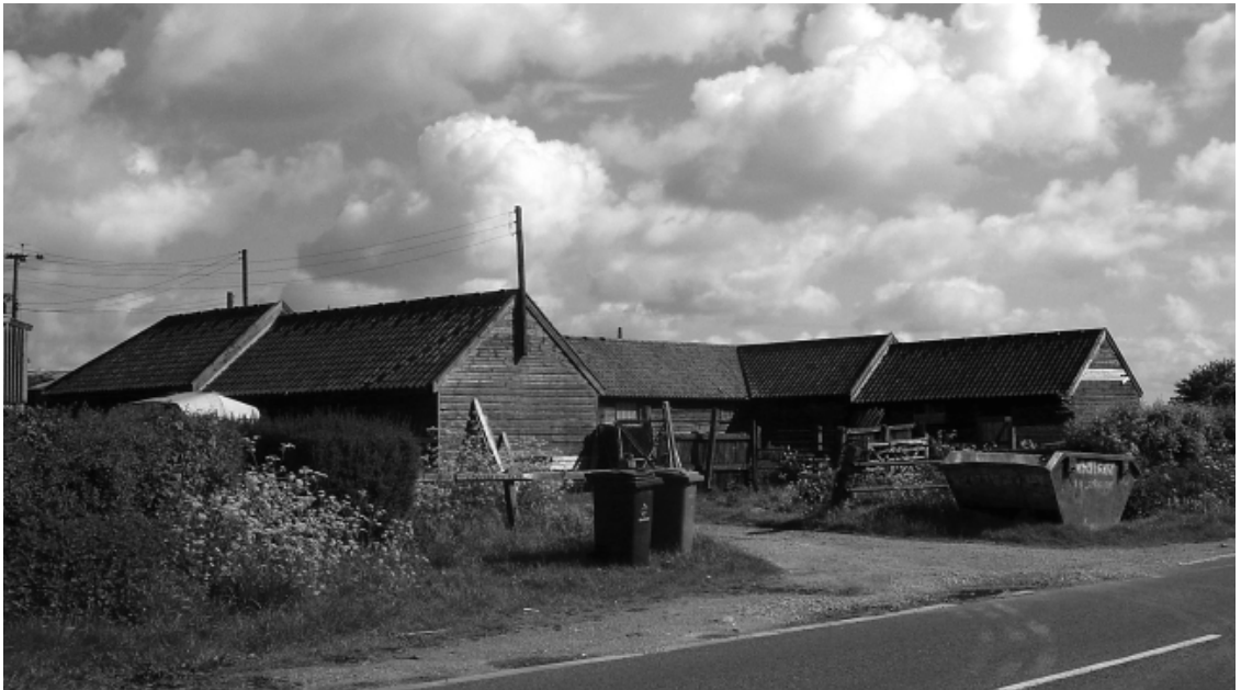
FIGURE 4. House and buildings at Oaklands (now Jubilee) Farm, Litcham.
