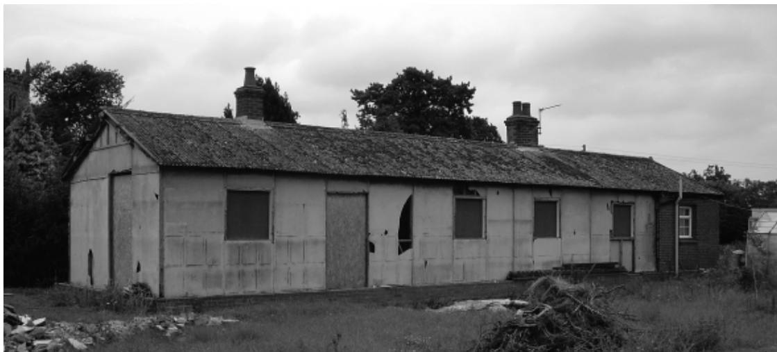
FIGURE 1. Asbestos bungalow in the process of demolition at Lingwood, on the Burlingham estates
