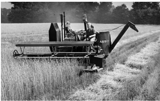
Early Massey Harris tanker combine with bat reel, 1947 Image: The Museum of English Rural Life, University of Reading.
