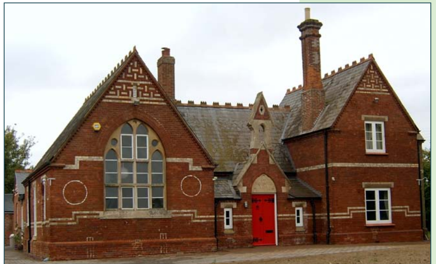
The U-plan Board school at Bracon Ash is typical of the 1870s, with ornate central entrance. The teacher's house forms one wing, the school room the other with a small class room in the centre.
